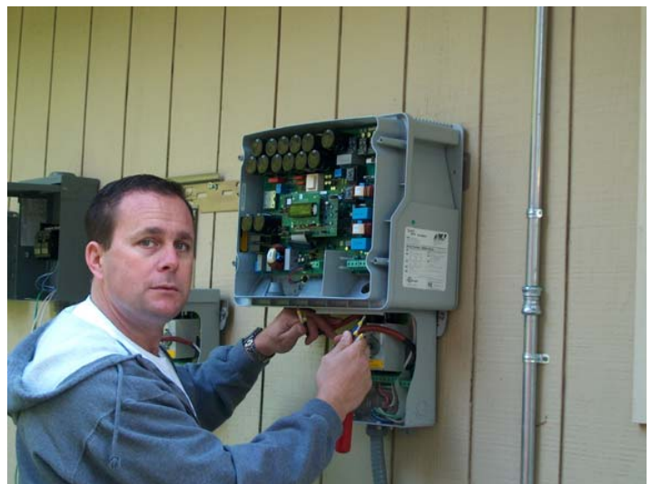
Eric Keith installs an inverter
